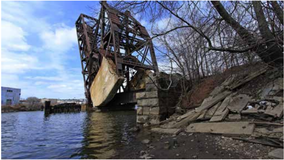
FIG. 11. Annie Bridge , a bascule bridge with concrete counterweight near Newark NJ.
